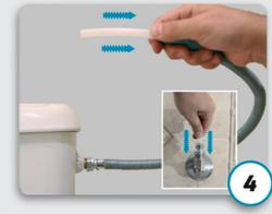
Insert the main pipe to the corrugated one and connect one end of the main pipe with the angle valve. Push the corrugated pipe so that there is a sufficient length of the main pipe to be connected with the speed fit until hearing the characteristic click.
