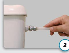
Push the pipe into the angle valve speed fit until you hear the characteristic click of successful connection.
