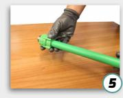
Joint them immediately without rotating until the marked welding depth is covered
